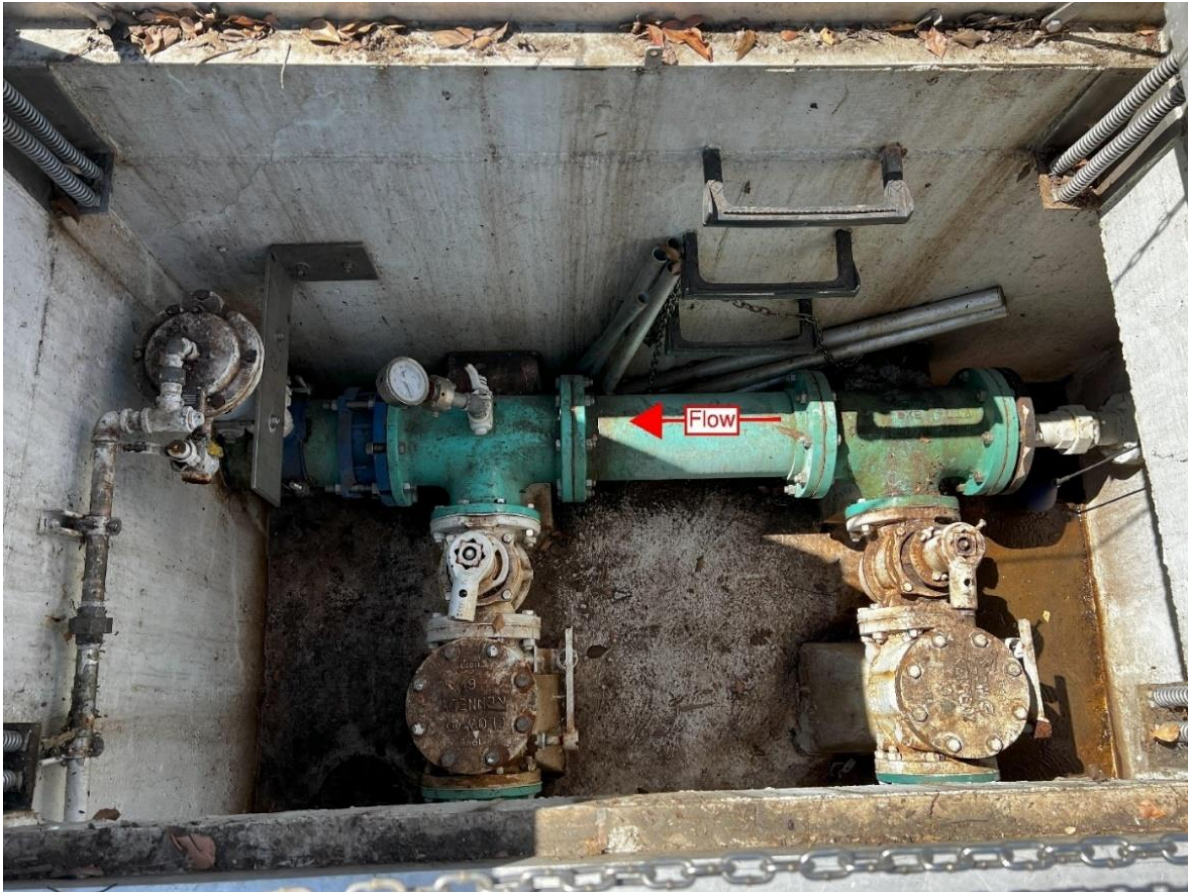
Figure 6. Scottsdale Pump Station Existing Pipe Configuration
