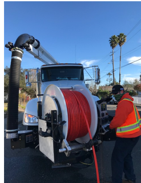
Crewmember Nate Adams conducting line cleaning operations
