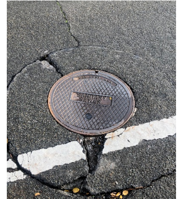
Broken collar on manhole, Virginia Ave., repaired by District contractor.
