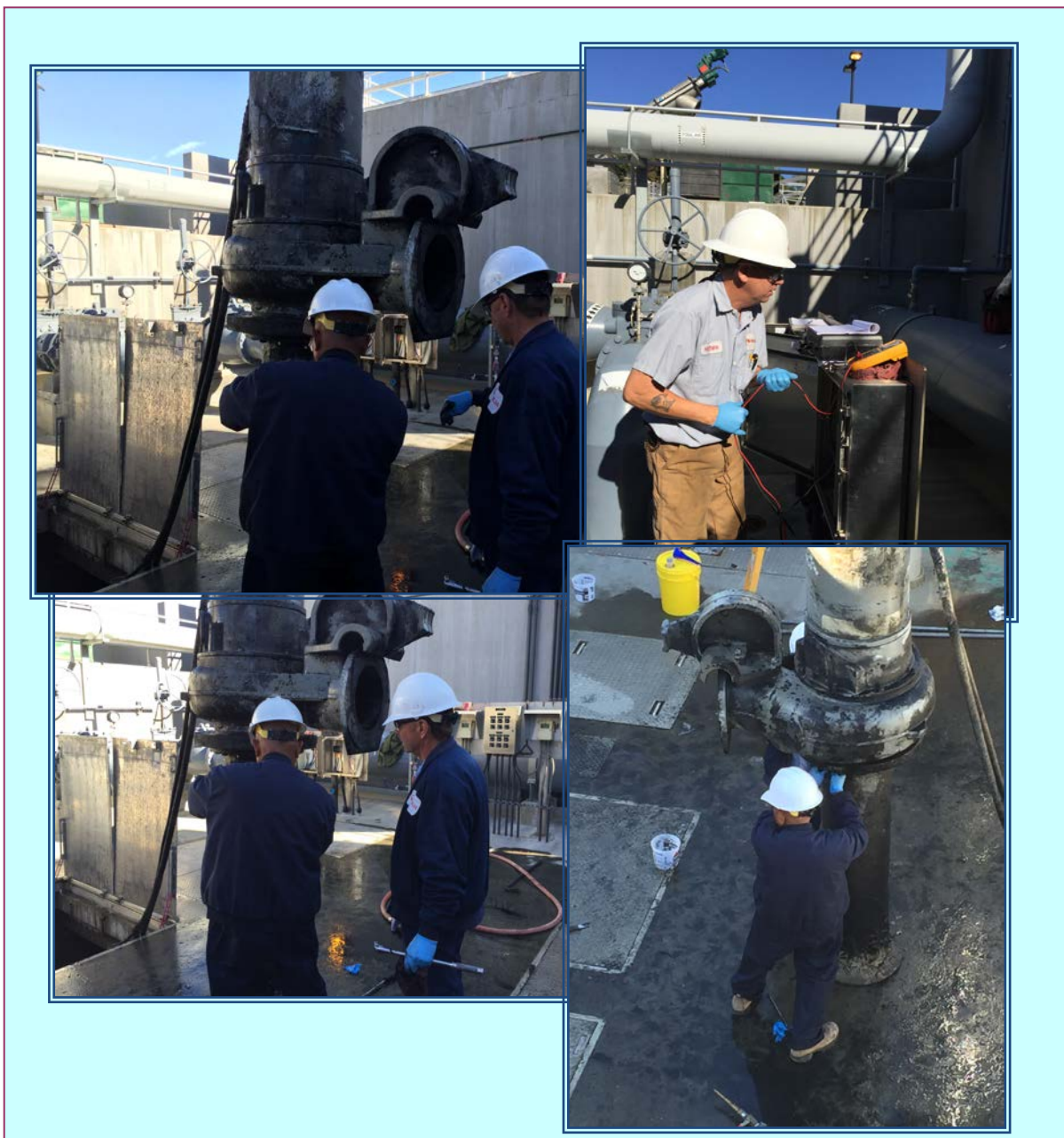
Jeff Hendricks, Alejo Cuntapay, and Matt Nausin perform annual manufacturer recommended inspection and maintenance on influent pumps.
