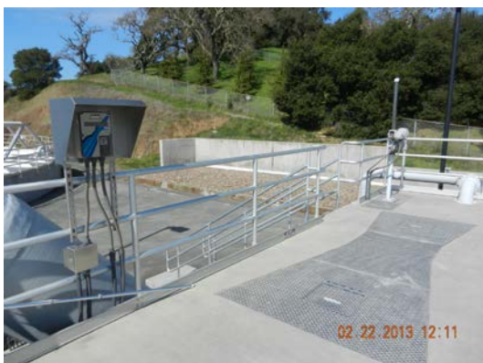
Above Left – Hydro Ranger level meter, hourglass shaped plating over Parshall Flume
