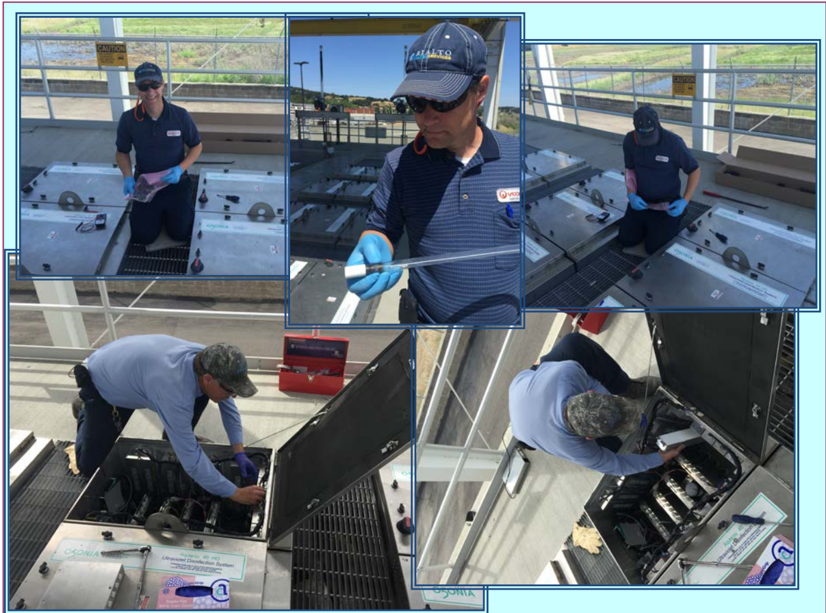
Replacement of Lamps and Ballasts on Ultra Violet Disinfection System
