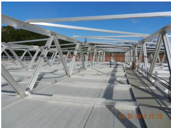
Above Left – Primary Clarifier #2, Superstructure supports the cover.
