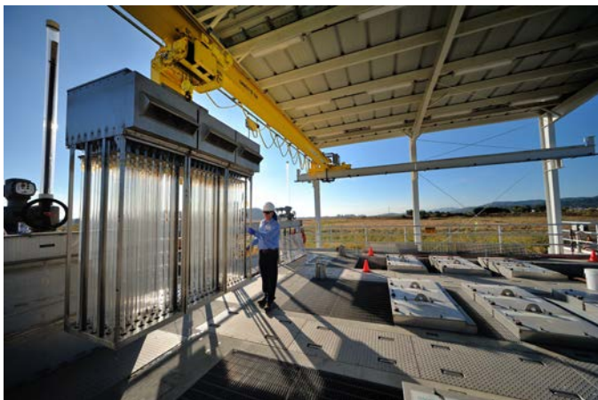
Left – UV Rack Removed for Cleaning Below – Preparing UV Rack for Removal
