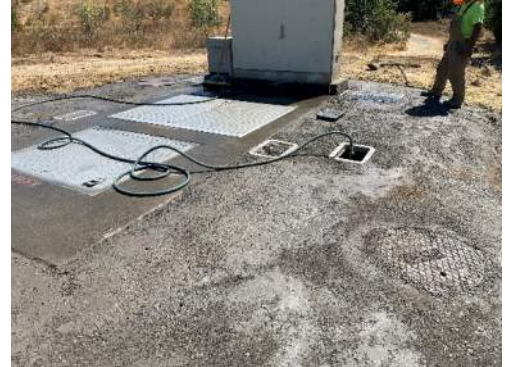
1. Contractor resurfacing and re-setting the boxes at Bahia 2 Pump Station
