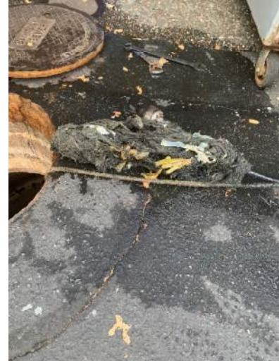
Root ball pulled from a siphon on Redwood Blvd.
