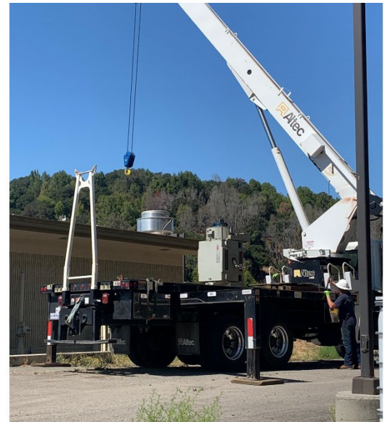
400 HP motor removal operation from Pump #3 at Irrigation Pump Station.
